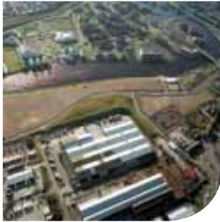
An aerial view of the site.
